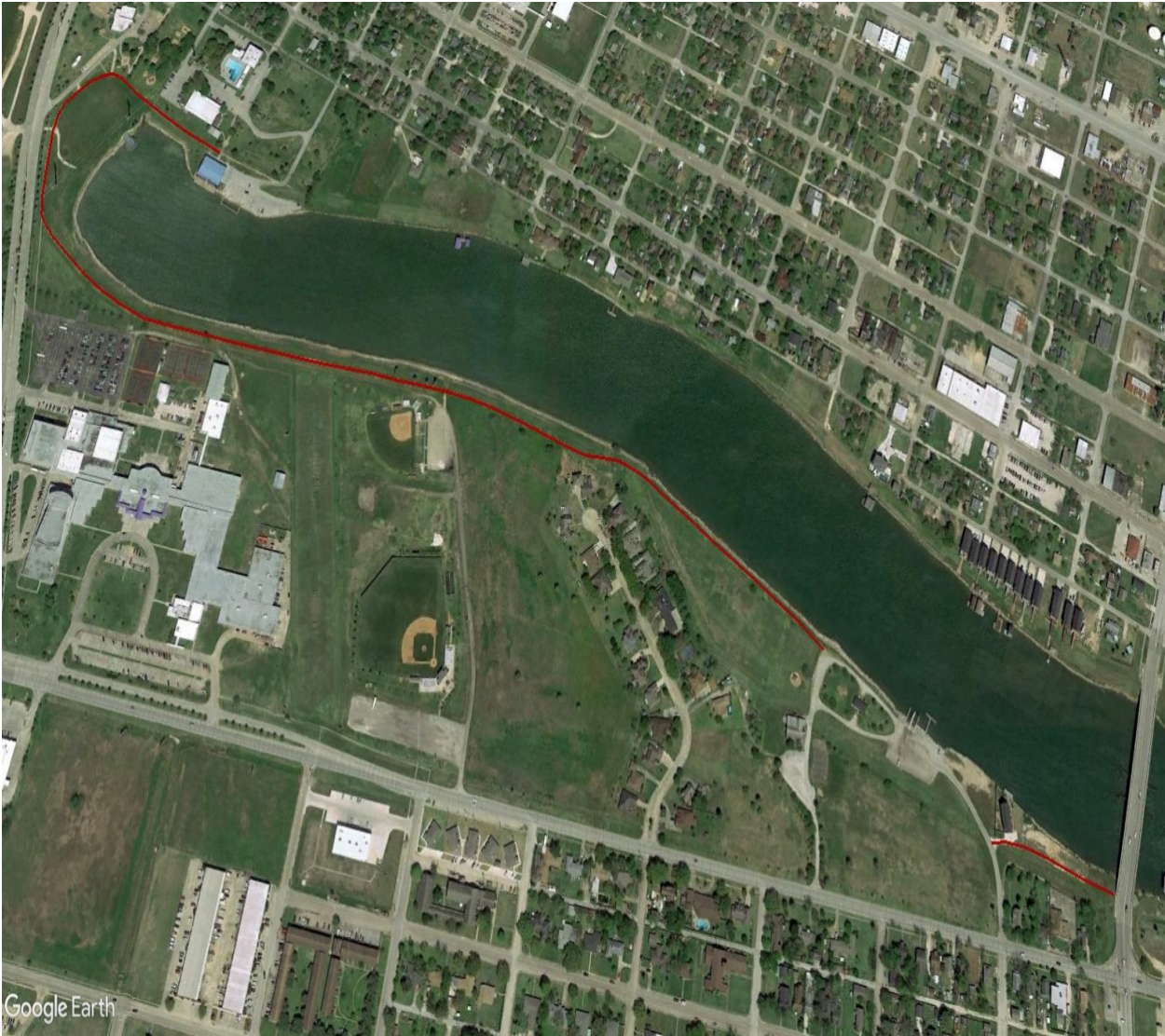
The project is 6 feet wide, and 1.8 miles in length to include ribbon curbs
